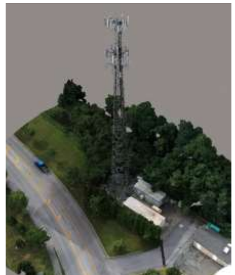
Cell tower inspection with photogrammetry and a 3D model.
