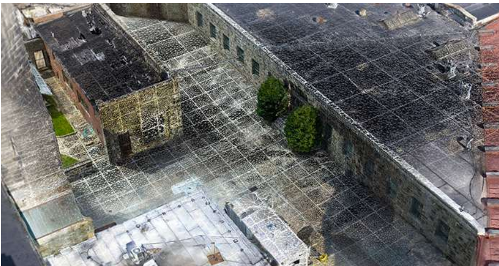
3D Model of a local landmark used for capital project planning. Aerial and still photography were used.
